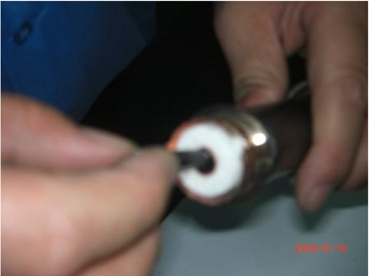
Clean inner conductor of swarf after tapping using adhesive tape or brush or similar
