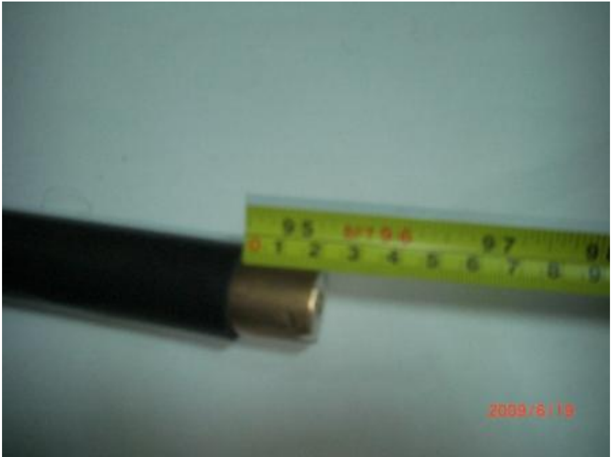
Leave 20mm of outer shielding
