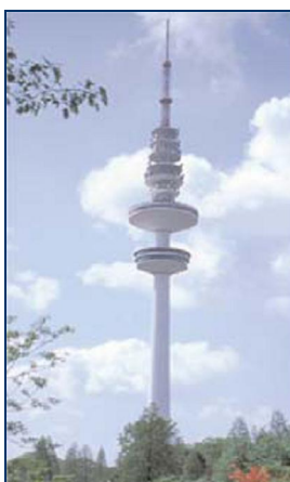
Stone-age technology: Thousands of these broadcast towers are in operation.
